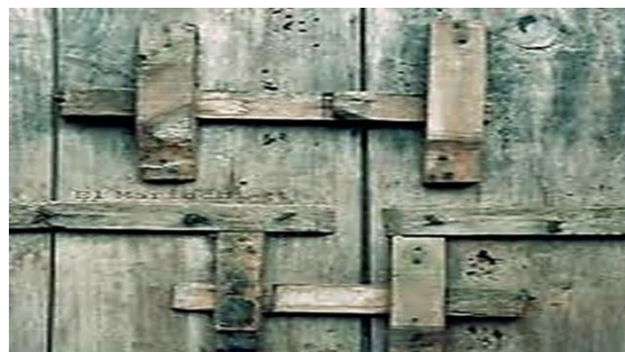
Image (illustration). A simple Latch 14 for locking a door of the emergency exit from inside your house
