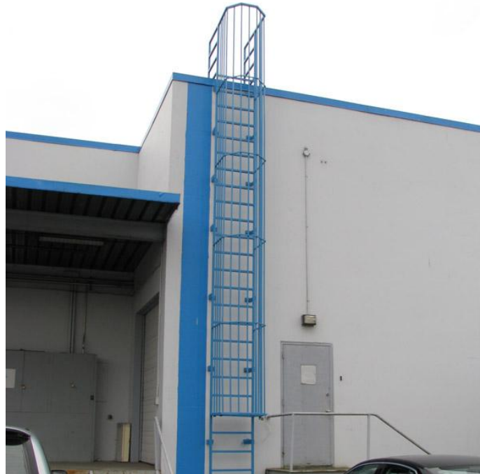
Image. The emergency exit with an OUTSIDE LADDER for you to climb up the roof in order to avoid a tsunami (illustration) 16 You can use a simpler ladder instead.
