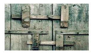
Image (illustration). A simple Latch<sup>14</sup> for locking a door of the emergency exit from inside your house
