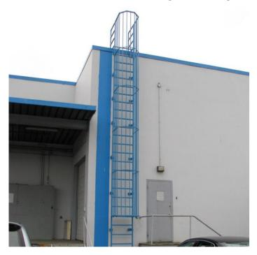
Image. The emergency exit with an OUTSIDE LADDER for you to climb up the roof in order to avoid a tsunami (illustration) <sup>16</sup>
